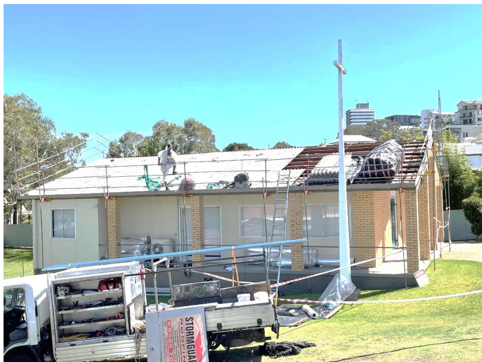
Replacement of old Asbestos Roof 2023
